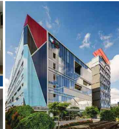
Building façade underwent a major facelift to achieve a modern look
